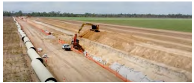
HAUGHTON PIPELINE STAGE 2
