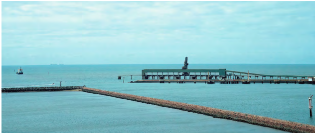
PORT OF TOWNSVILLE - CHANNEL UPGRADE
