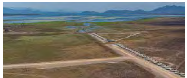
HAUGHTON PIPELINE STAGE 1
